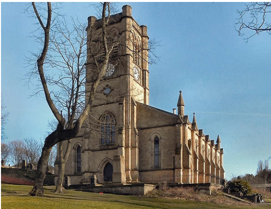
Fig. 47.1 St. Peter's Church, Blackley, UK. Designed by E. H. Shellard, ca. 1845. The church has the basic form of a Greek temple but is dressed up with Gothic features such as pointed windows and superfluous buttresses. Photo by David Dixon
